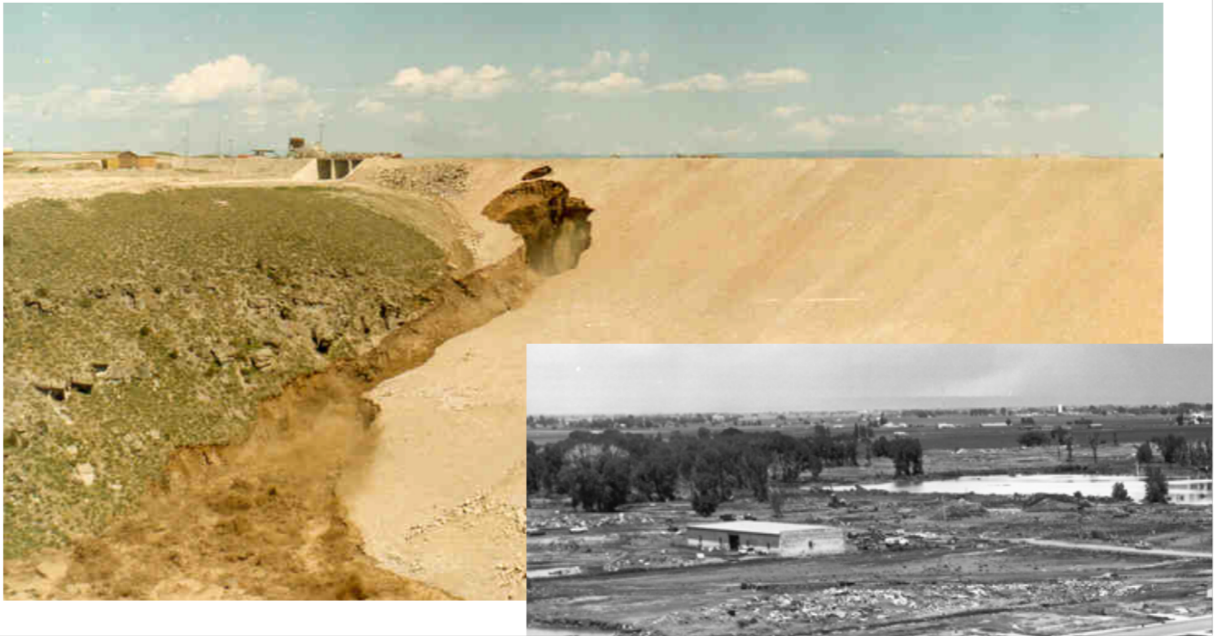
8 minutes before dam failure
