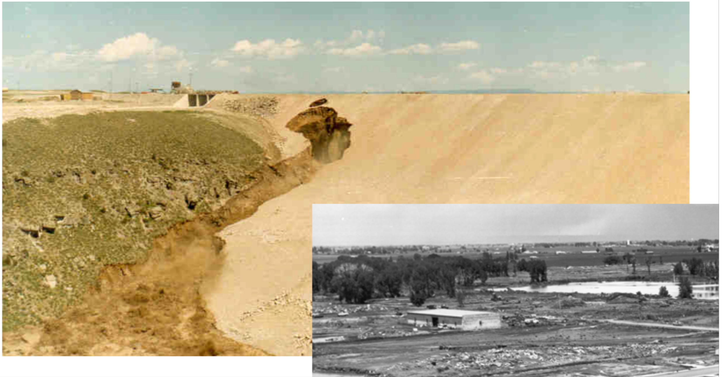
8 minutes before dam failure
