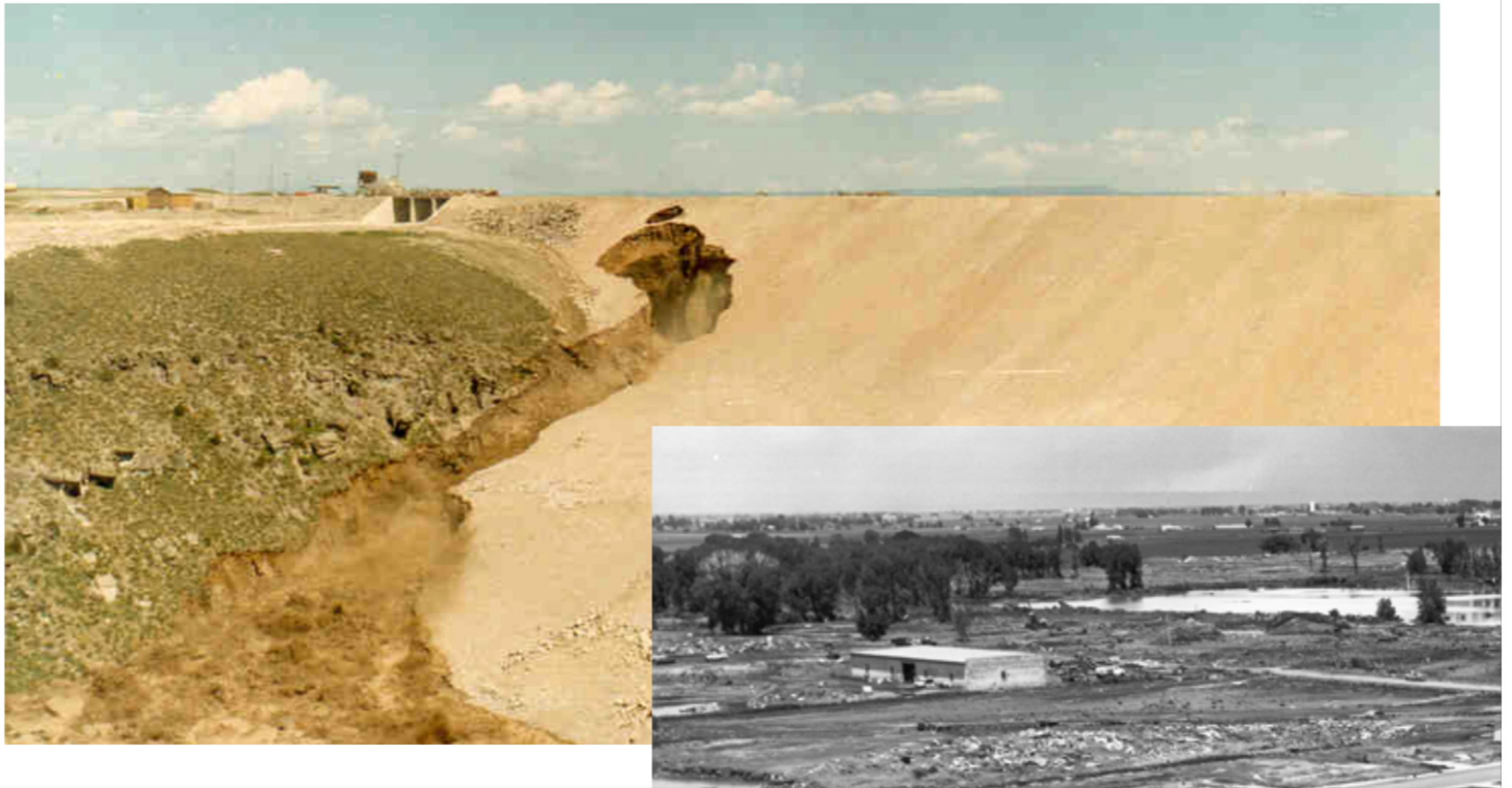
8 minutes before dam failure
